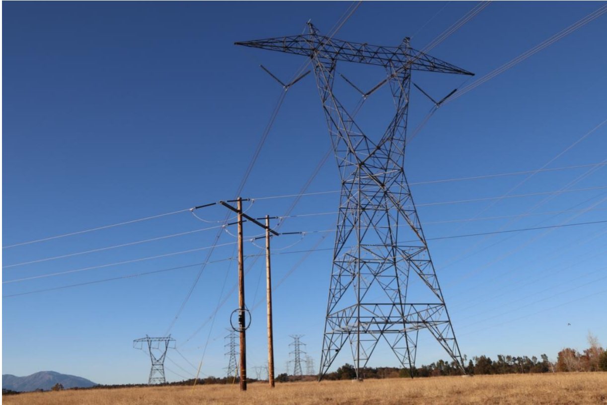
Figure 16. Image of the 115 kV transmission line connecting the Cottonwood Substation to the Humboldt Substation via Bridgeville as it passes under a 500 kV line near Cottonwood.
