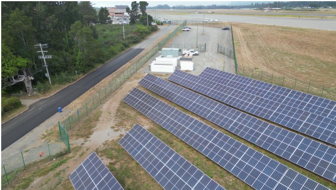
Figure 14. Aerial photograph of the solar array, battery, and switchgear equipment of the Redwood Coast Airport Microgrid (RCAM). Source: Photograph by Greyson Adams, August 2023.
