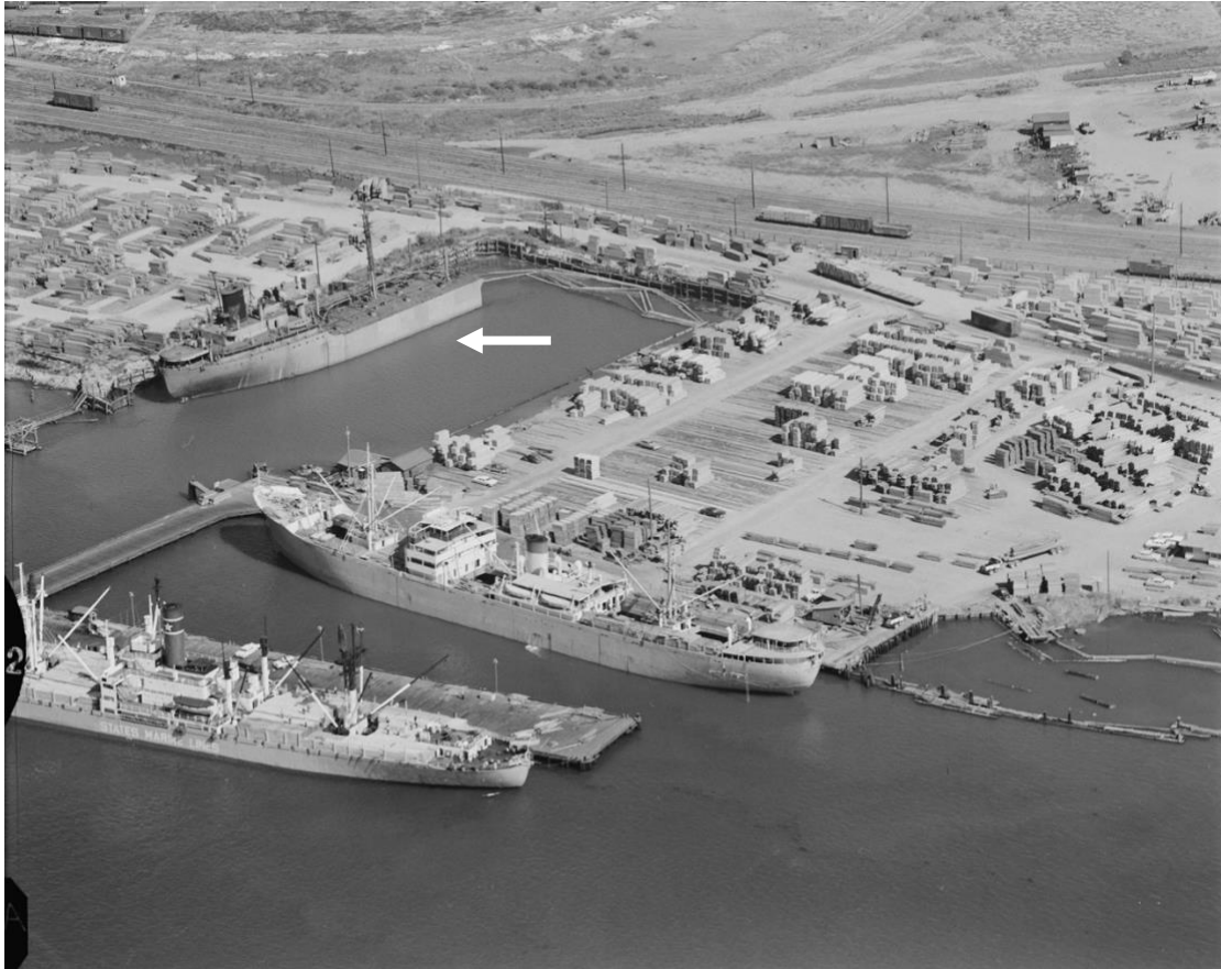
Figure 3. Aerial photograph of the Donbass III, the vessel that served as a 5 MW power plant from 1947 to 1958. The Donbass III is the half vessel facing away from shore in the left side of the image. A white arrow indicates its location. Source: Photo ID 2001.01.2277, Shuster Aerial Photograph Collection, Cal Poly Humboldt Library. Photo date: August 15, 1957.
