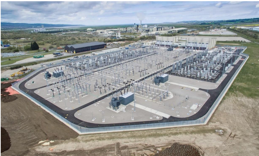
Figure 3 - Example LCC Converter Station (Western Link, 2200MW)
