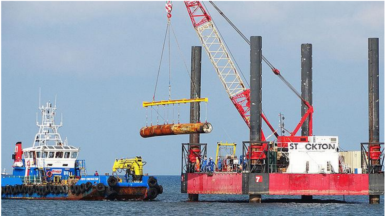
Figure 14. Example of Direct Pipe® at Beatrice Offshore Wind Farm with Marine Support https://www.herrenknecht.com/en/references/referencesdetail/beatrice-offshore-wind-farm-landfall/
