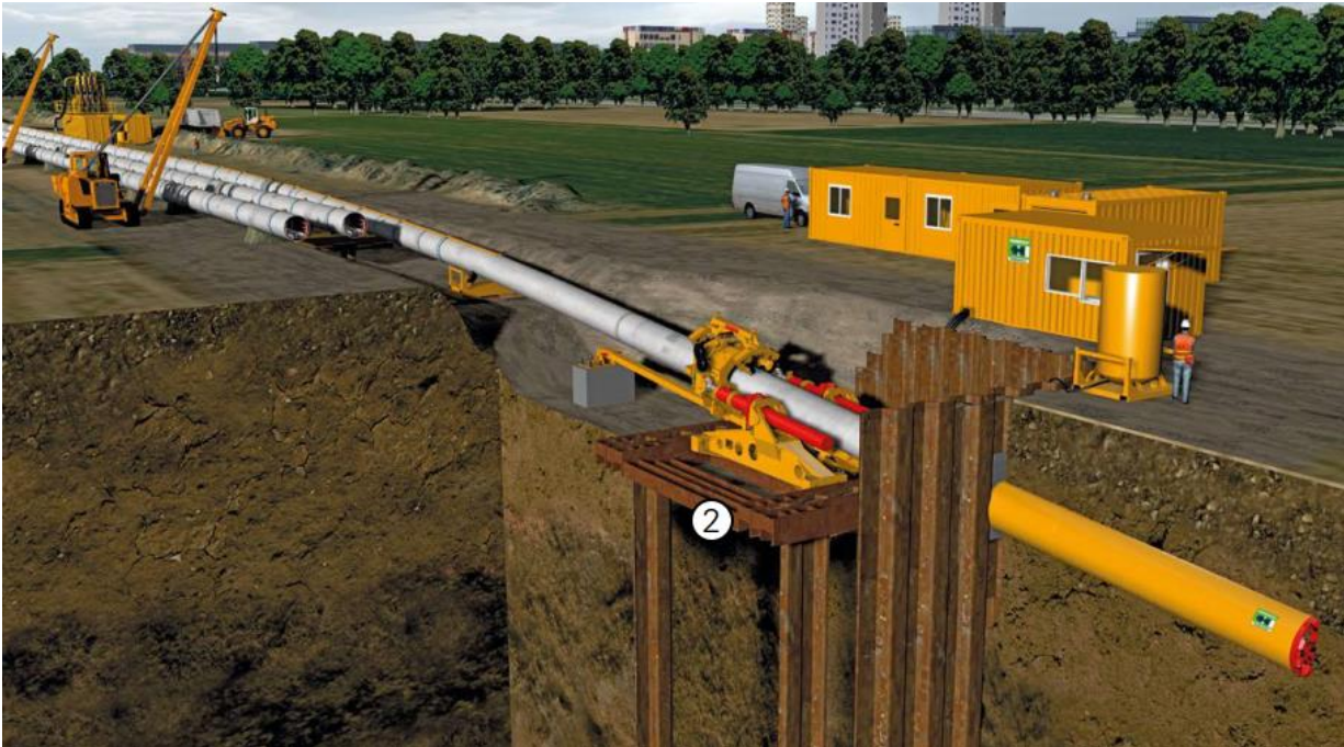
Figure 12. Direct Pipe® Process
