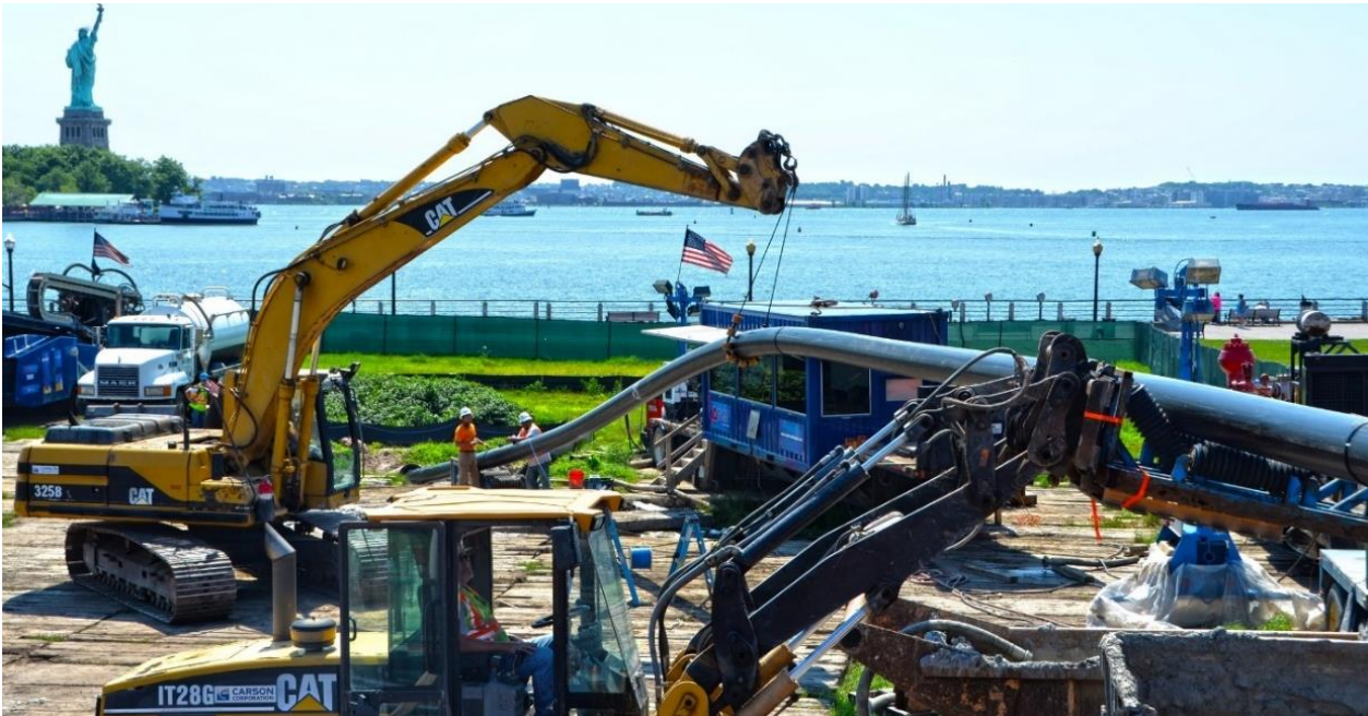
Figure 9. Example HDD Installation Workspace - Liberty Island Water/Wastewater (Mott MacDonald)
