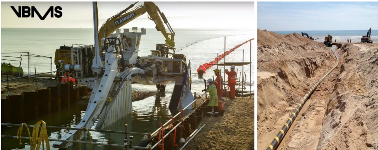
Figure 15 - Trenched Cable Landing Concept Examples: Plough (left) and open cut trench (right)
