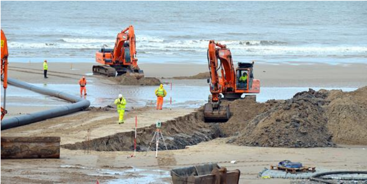
Figure 16. Example of Beach Works Around Cable Landfall (Walney Offshore Wind Farm)
