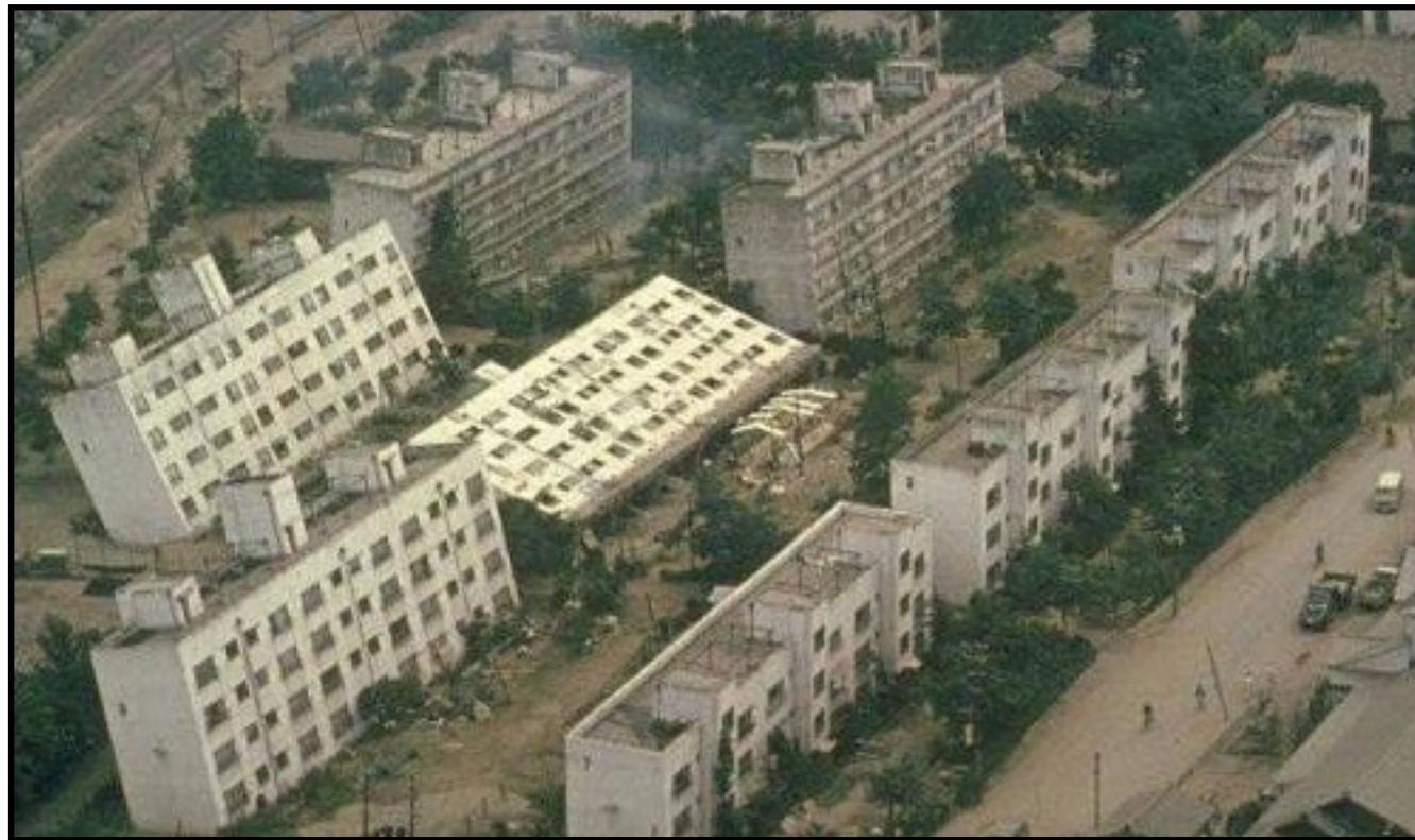
Liquefaction-induced collapse of buildings in Niigata, Japan during 1964 M7.6 event (Wikipedia)
