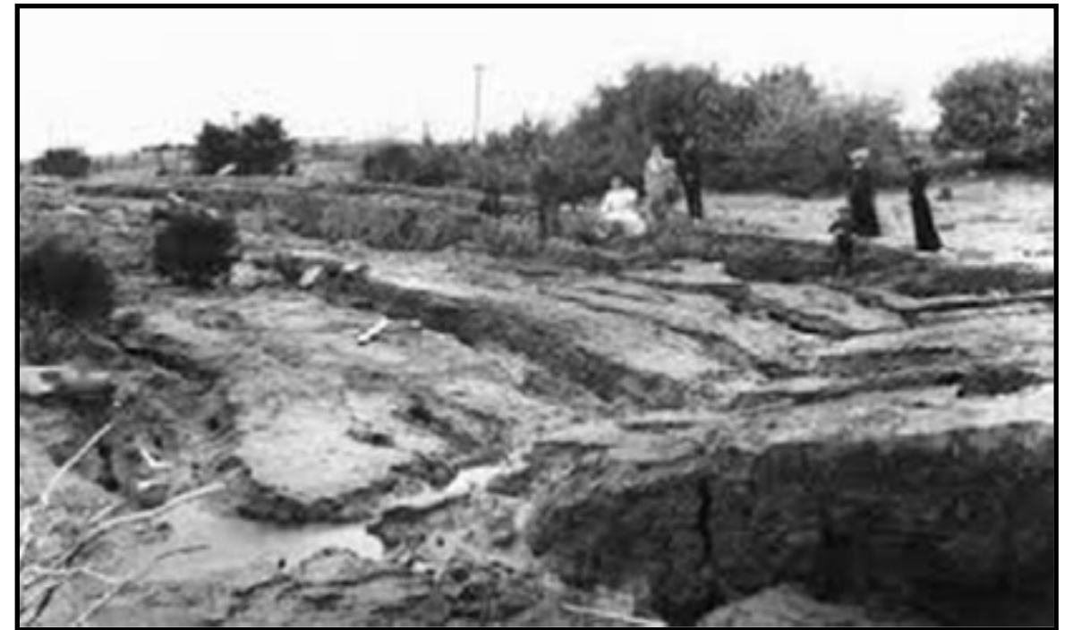
Liquefaction-induced lateral spread at Port Kenyon, lower Eel River, formed during 1906 earthquake (From Dengler, 2008)
