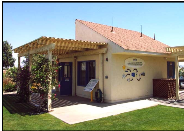
Figure 9. Interpretive signs at the Schatz Hydrogen Generation Center at SunLine Transit Agency in Thousand Palms, CA.
