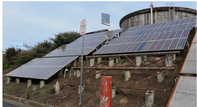
Fig. 1. A view of the array during decommissioning after two subarrays had already been removed (Photo Credit: Mark Rocheleau)
