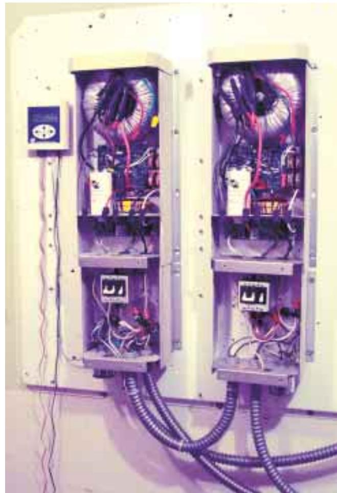
**Advanced Energy's AM100 Inverter Monitor (left) and the interior of the GC-1000 inverters.**
