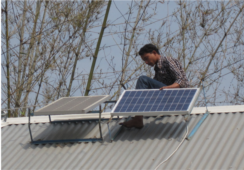
Fig. 3c. In Bangladesh, installing a solar module for a solar home system on a roof (photo: A. Jacobson).
